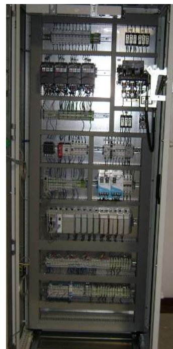
Floor standing industrial control panels
